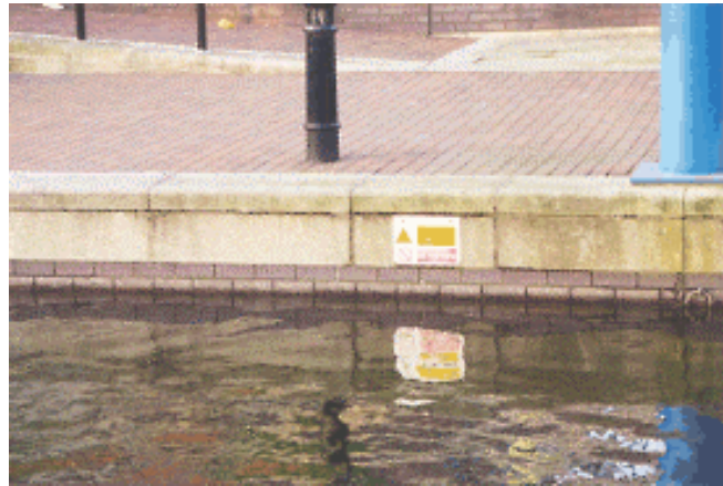
Band 1 solution - Well defined edge using a coping stone plus bollards
